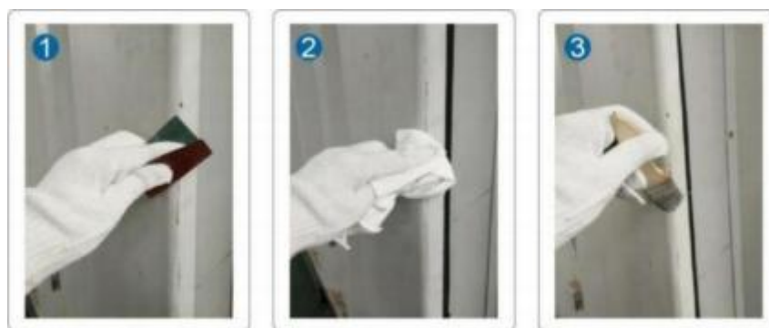
picture 9-38 Sanding and paint repair diagram
